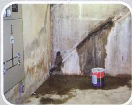
CRACK REPAIR DAY TWO
