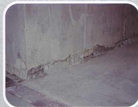
COLD JOINT REPAIR — AFTER
