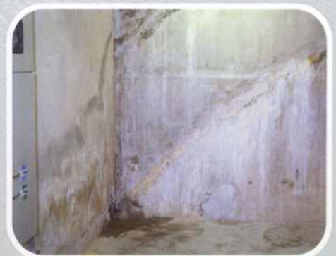
CRACK REPAIR DAY SEVEN
