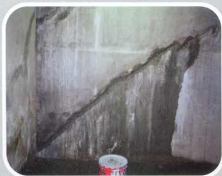
CRACK REPAIR DAY ONE
