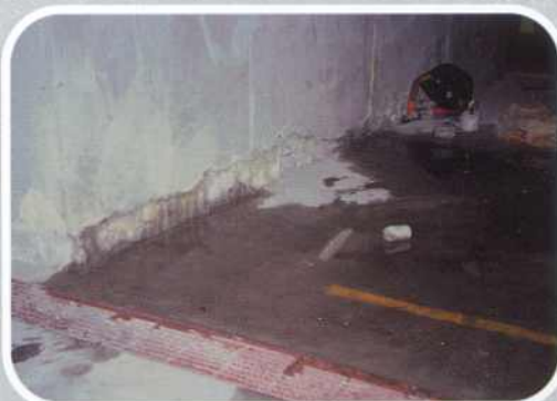
COLD JOINT REPAIR — BEFORE
